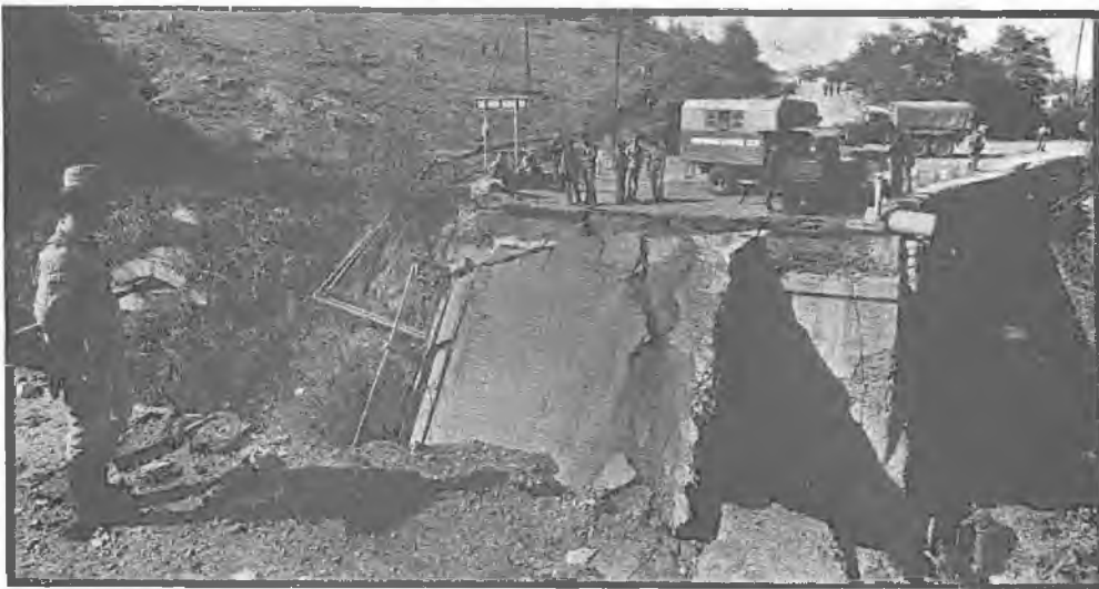
War on the roads. The bridge across the road Shusha-Agdam.
