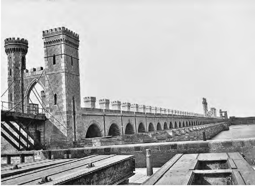
Delta Barrage. This dam was built by French engineers for Mehmet Ali to control the flow of Nile waters into the Rosetta and Damietta branches of the Nile and thus to facilitate the perennial irrigation of the Nile Delta. It soon developed leaks, which British engineers repaired during the Cromer era. (Library of Congress)
