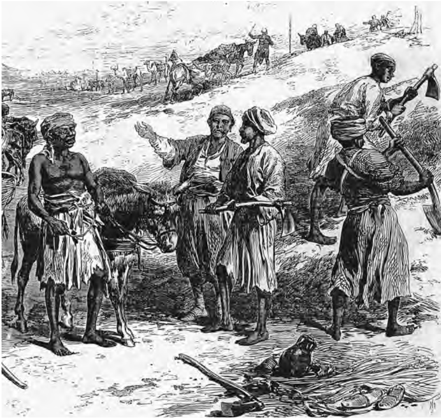
Hired Egyptian workers and their donkeys remove earth from the future bed of the Suez Canal in early 1869. Although dredging machines had replaced unpaid peasant laborers for most excavation work, human labor was still needed as the deadline for completing the canal drew near. (Illustrated London News, March 13, 1869)
