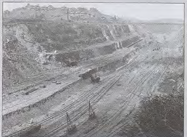
The building of the Panama Canal.
