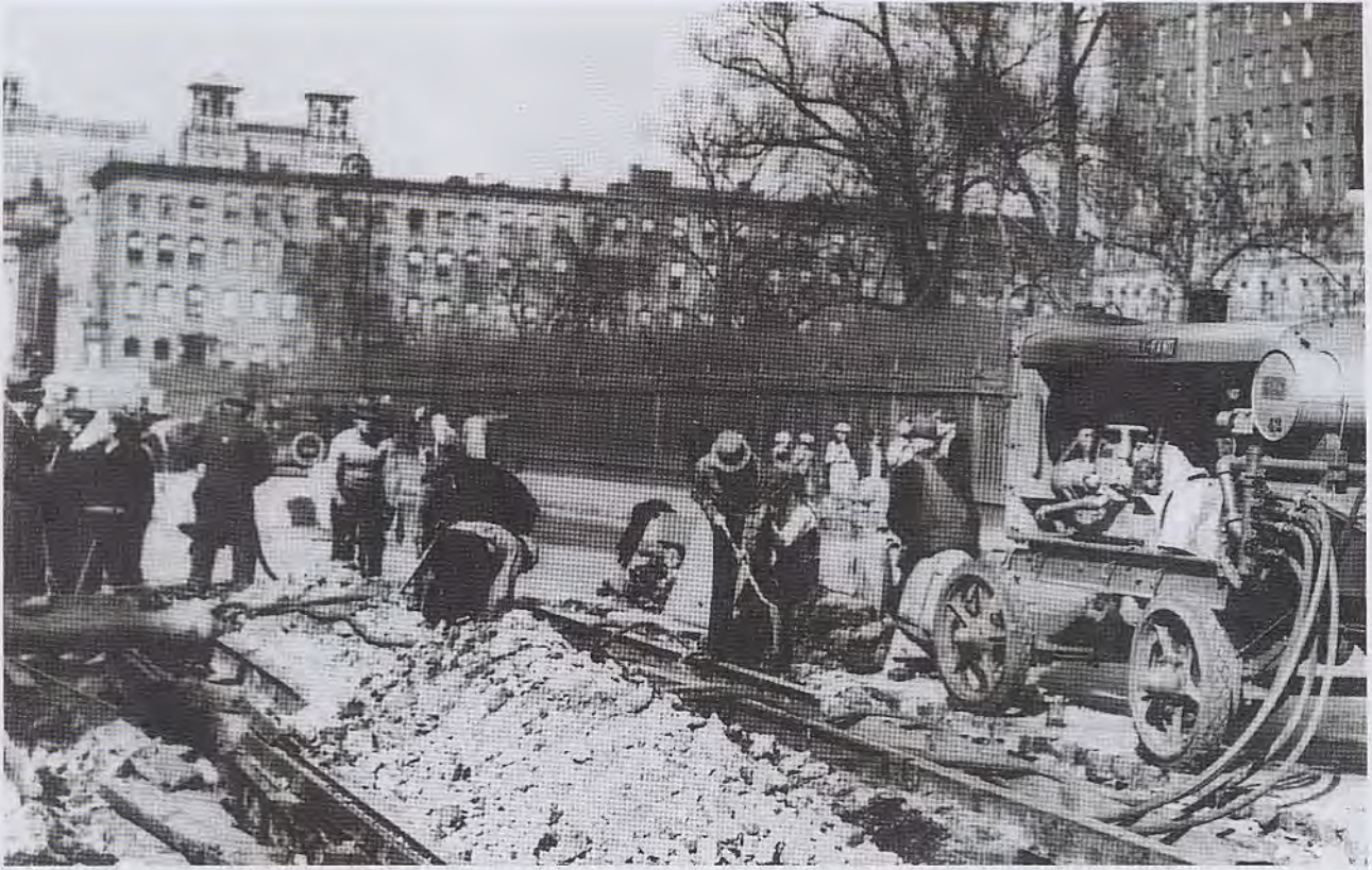
Workers on a W.P.A. project in the middle of the 1930s.
