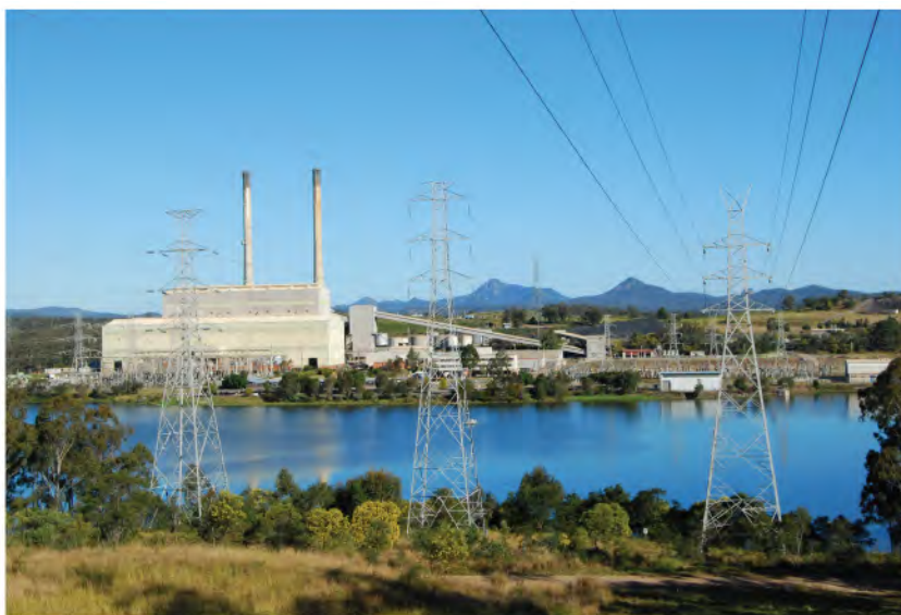
Figure 18.42 (a) Schematic of an electrostatic precipitator. Air is passed through grids of opposite charge. The first grid charges airborne particles, while the second attracts and collects them. (b) The dramatic effect of electrostatic precipitators is seen by the absence of smoke from this power plant. (credit: Cmdalgleish, Wikimedia Commons)
