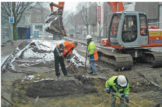
Fig. 2 Excavation in de Gerard Noodtstraat in the centre of Nijmegen (Photo: Afra Koopman, BAMN)
