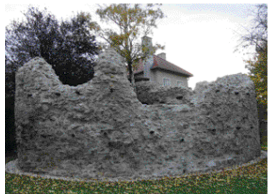
Fig. 4 The north-eastern fan-shaped tower, fort Zeiselmauer after conservation in 2007 (Photo: E. Kuttner)
