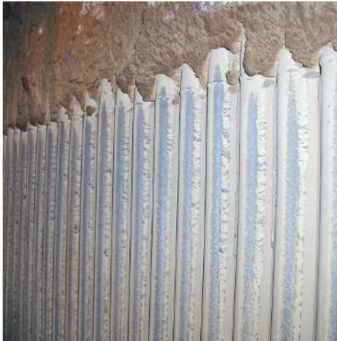
Adherences at the heat exchanger in power plants can be avoided through ceramic nanocoatings. Top: uncoated surface; bottom: with nanocoating (source: ItN Nanovation)
