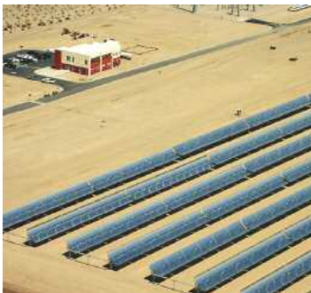
The 64-megawatt parabolic trough power plant "Nevada Solar One" in the US-state of Nevada, on stream since June 2007, supplies approx. 129 million kilowatt hours (kWh) of solar energy each year (source: Schott).
